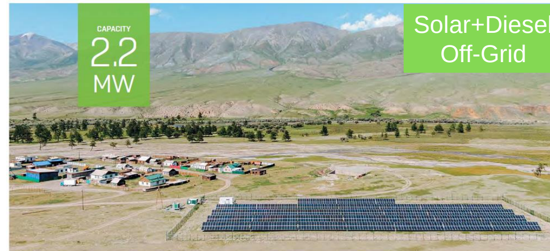
Republic of Tuva, villages of Mugur-Aksy and Kyzyl-Khaya (pop. 6,000) Stand-alone diesel-solar power plant
