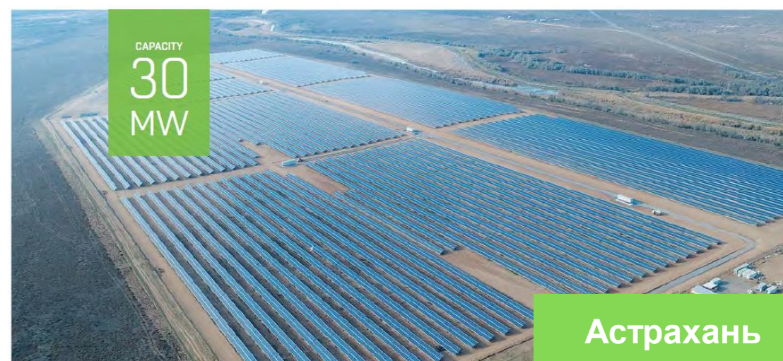
Limansky Solar Power Plant. Astrakhan Region
