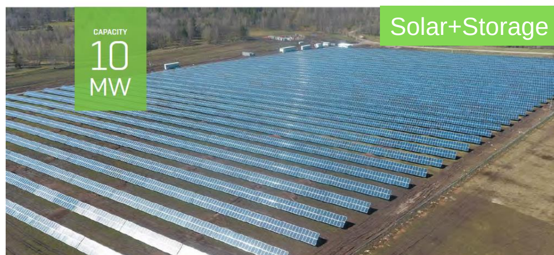
Burzyansky Solar Power Plant. Republic of Bashkortostan Russia's largest solar power plant with industrial energy storage
